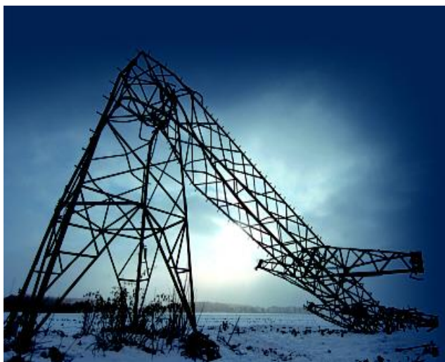
Figure 2.3: Collapse of a transmission tower.
