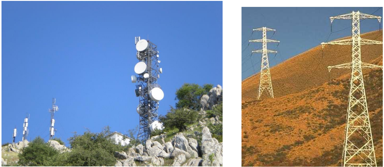
Figure 2.1: Lattice towers: telecommunication towers and transmission towers.
